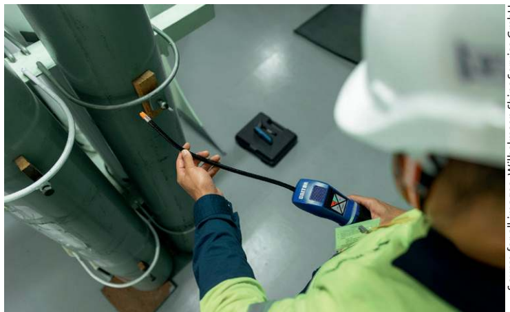
Figure 2: Engineer on board searching for refrigerant leaks with Unitor™ Refrigerant leak detector
