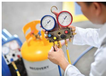
Figure 4: Refrigerant recovery in action
