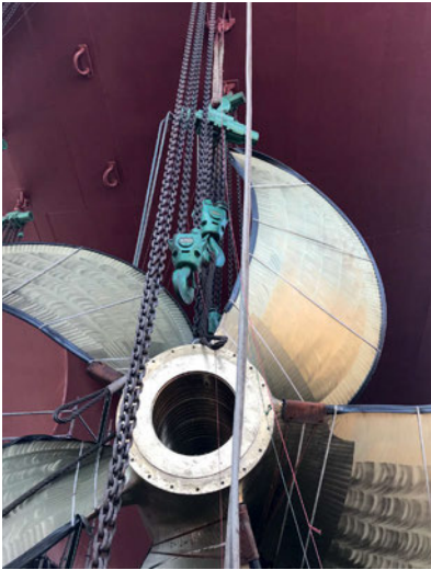
Ship propeller installation with JDN hoists in drydock
