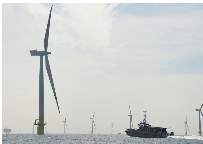
In Germany, the Federal Maritime and Hydrographic Agency (BSH) has now determined the suitability of further areas in the North Sea for the installation of offshore wind parks
