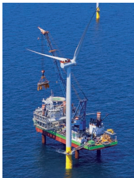
Calm weather conditions are to be favoured for the installation and maintenance of offshore wind parks
